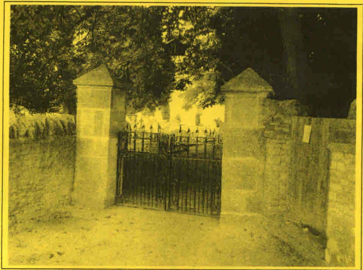
The repaired Memorial Gates
